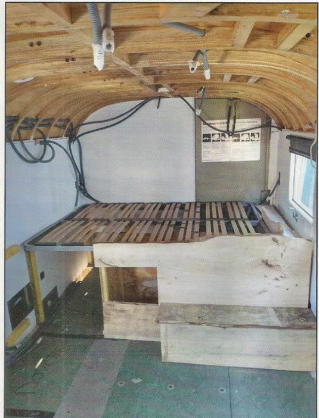
The bed being built in the rear of the truck.
